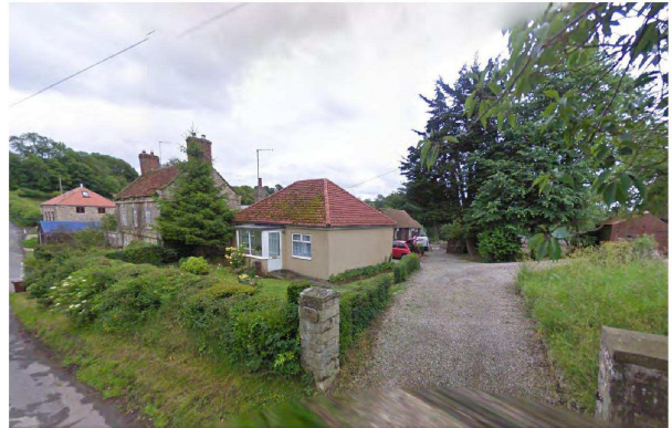
View of Acklam Lodge from Main Street, Looking South-east
